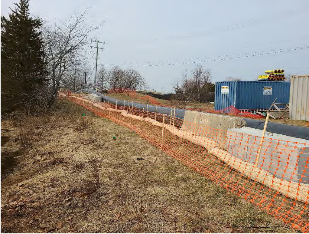
Photo 19. From the vicinity of the USACE Corps in the eastern portion of the pipeline replacement, looking west. (01-14-21)
