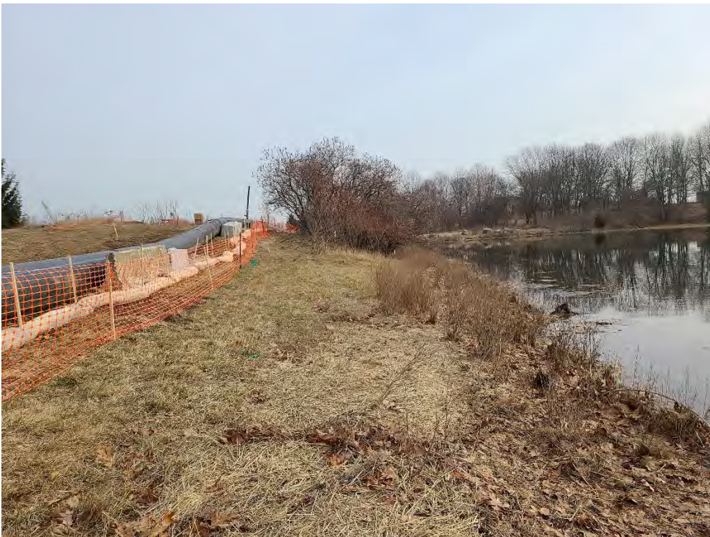
Photo 20. From the vicinity of the USACE Corps in the eastern portion of the pipeline replacement, looking east. (01-14-21)
