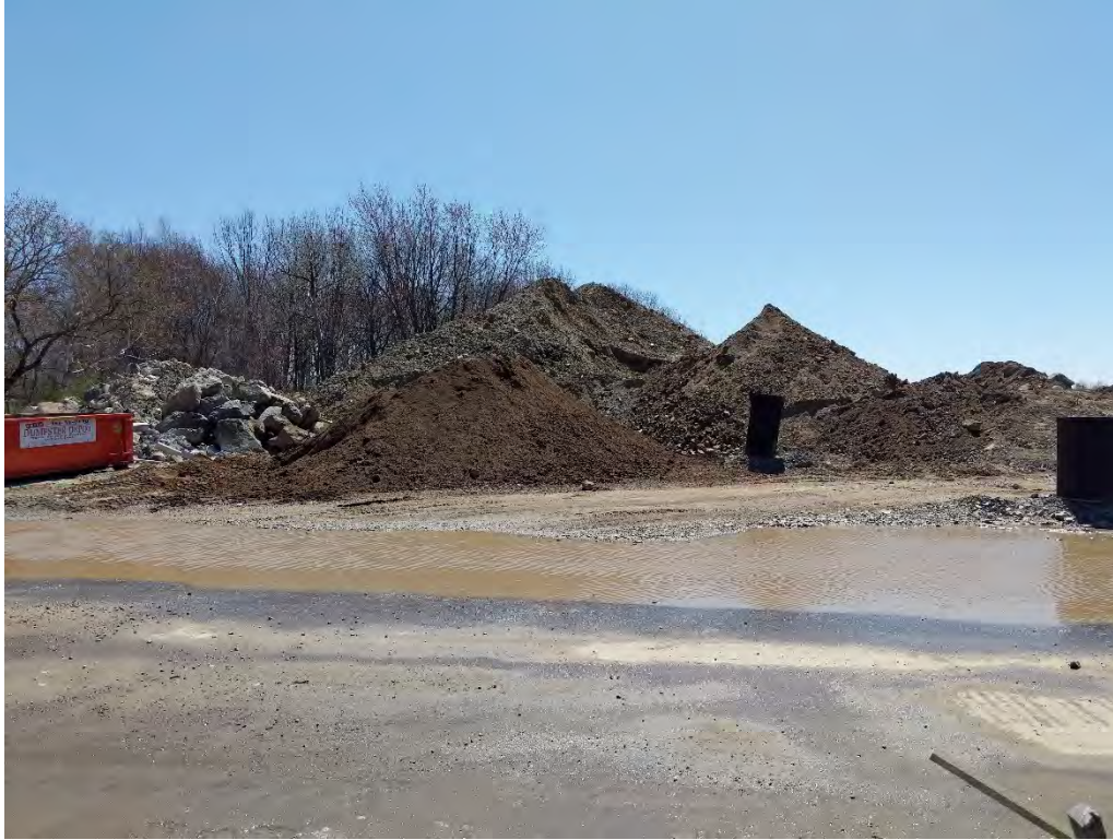
Photo 9. Spoil pile in construction laydown area at the proposed parking site, looking south. (04-23-20)
