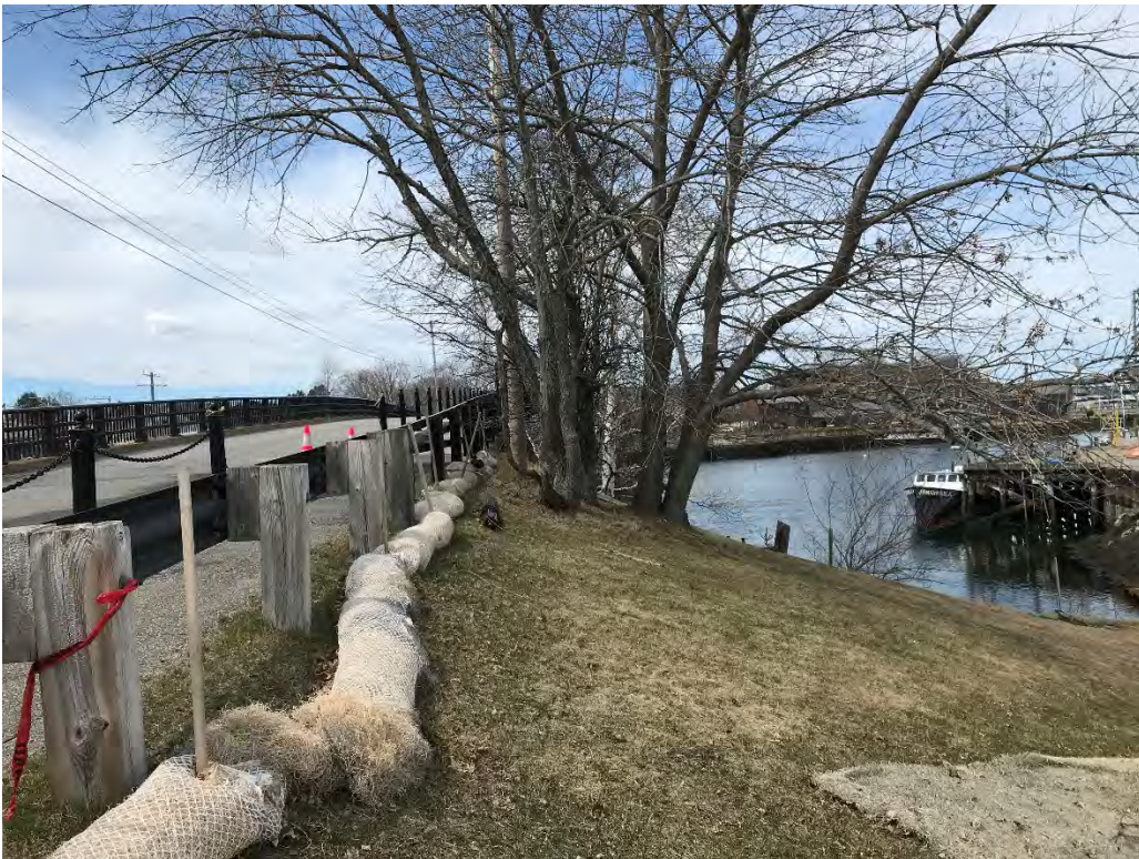
Photo 14. From northern embankment off east end of Peirce Island Road Bridge, looking west. (04-06-21)
