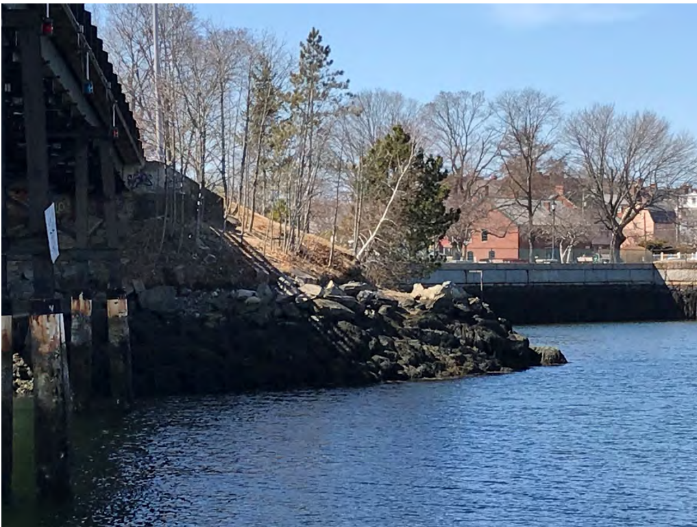
Photo 24. Shoreline off northwestern corner of Peirce Island Road Bridge looking west. (03-23-21)
