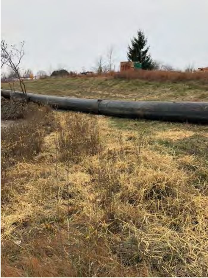
Photo 3: Staw Restoration in Area B
