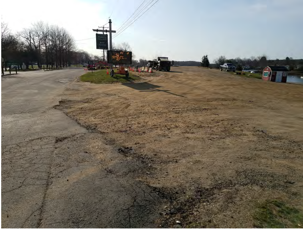
Photo 27. From the south side of the Peirce Island Road Bridge facing east. (04-15-21)
