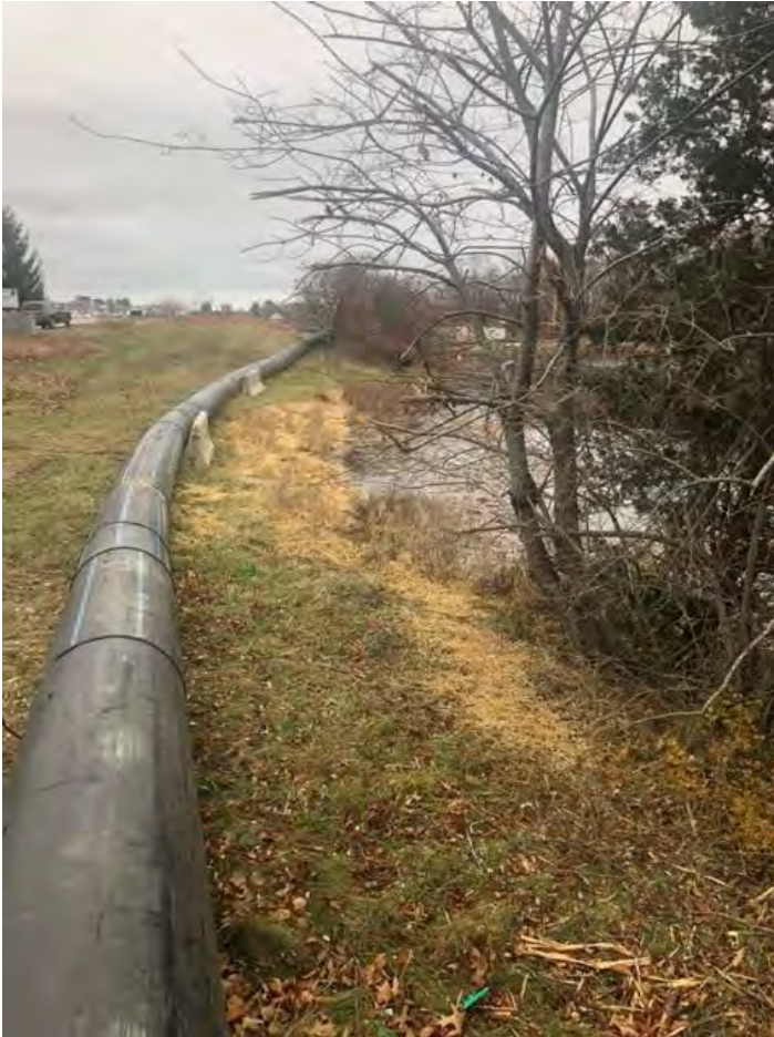
Photo 1: Straw Restoration at Area A
