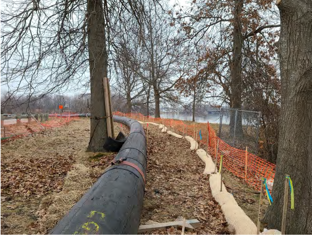
Photo 17. Along the pipeline replacement near Grid 42 of the tree inventory for the Pipeline Survey, looking east. (01-14-21)
