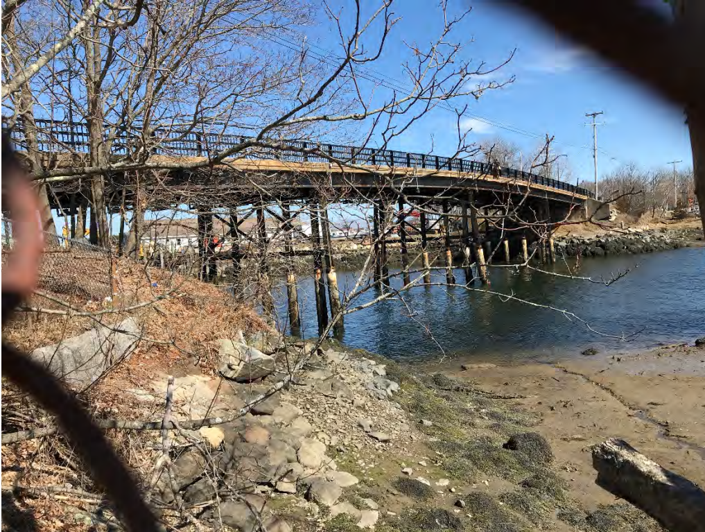
Photo 23. Shoreline off southwestern corner of Peirce Island bridge looking northeast. (03-23-21)
