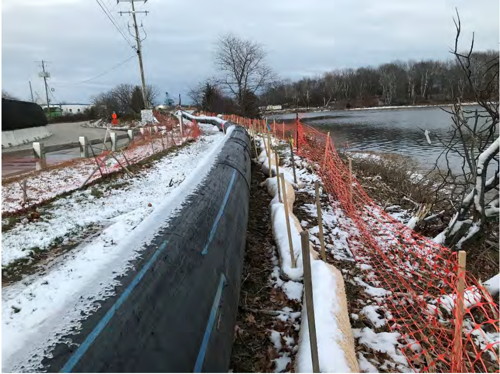
Photo 3: Construction Fencing Along the Length of Temporary Sewer Force Main
