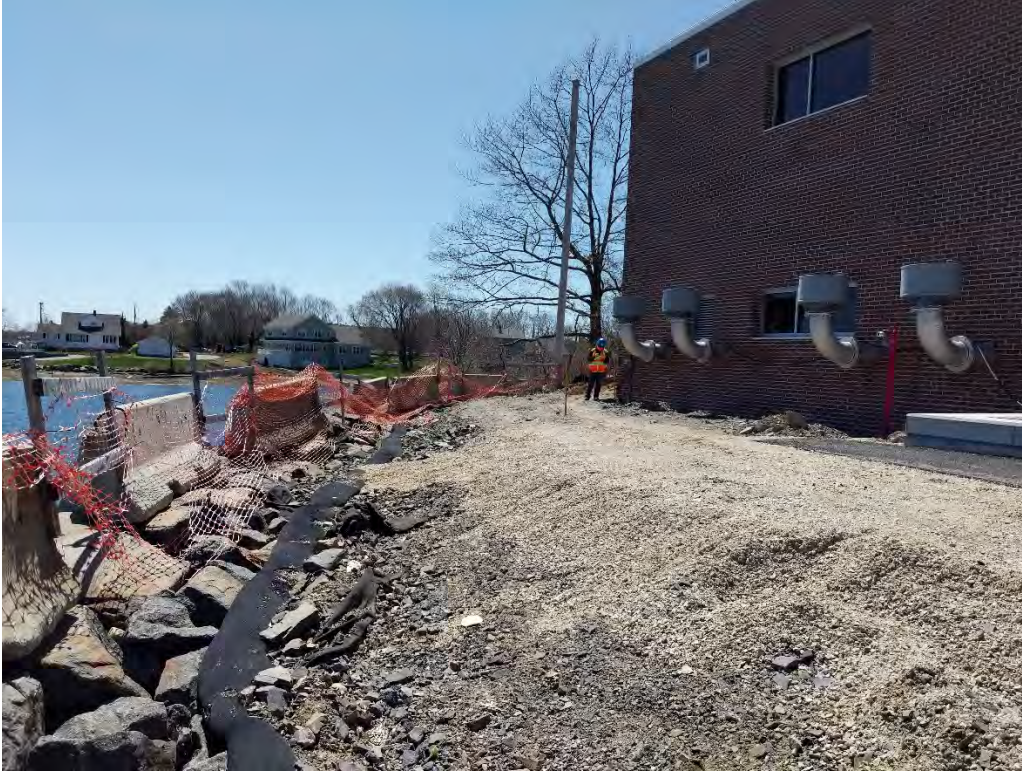
Photo 11. Southern end of the proposed path that curves around the southeastern corner of the wastewater treatment facility, bordered by rip-rap to the east, looking south. (04-23-20)
