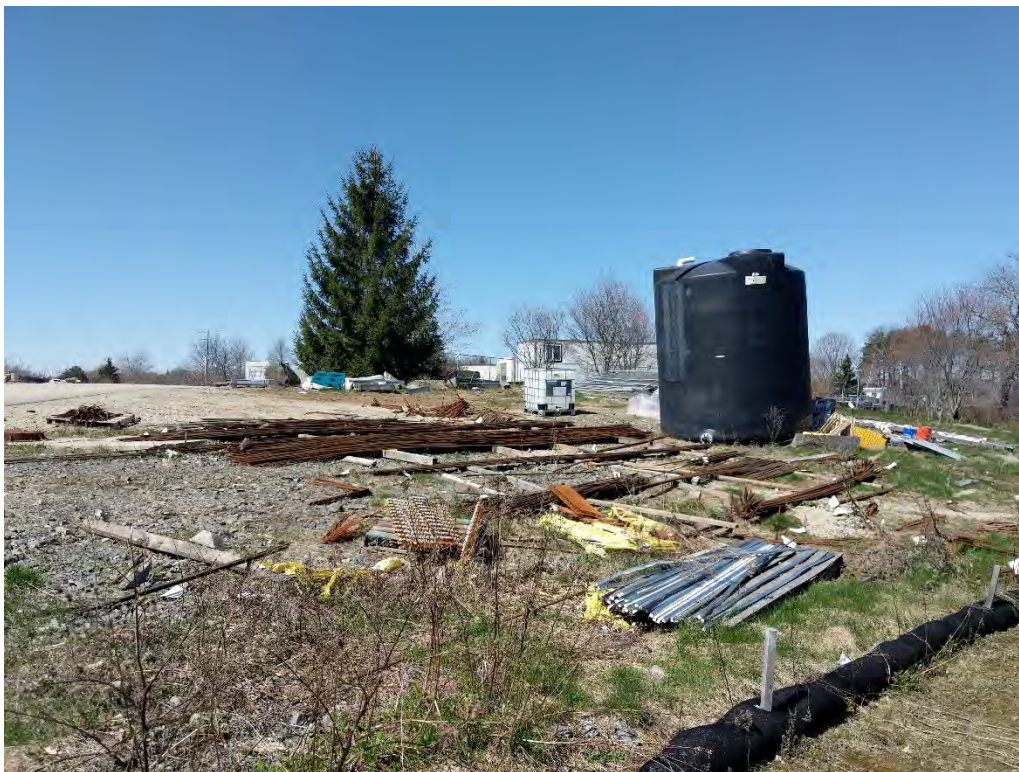
Photo 2. Construction laydown area in developed Tidal Buffer Zone, looking north from salt marsh. (04-23-20)
