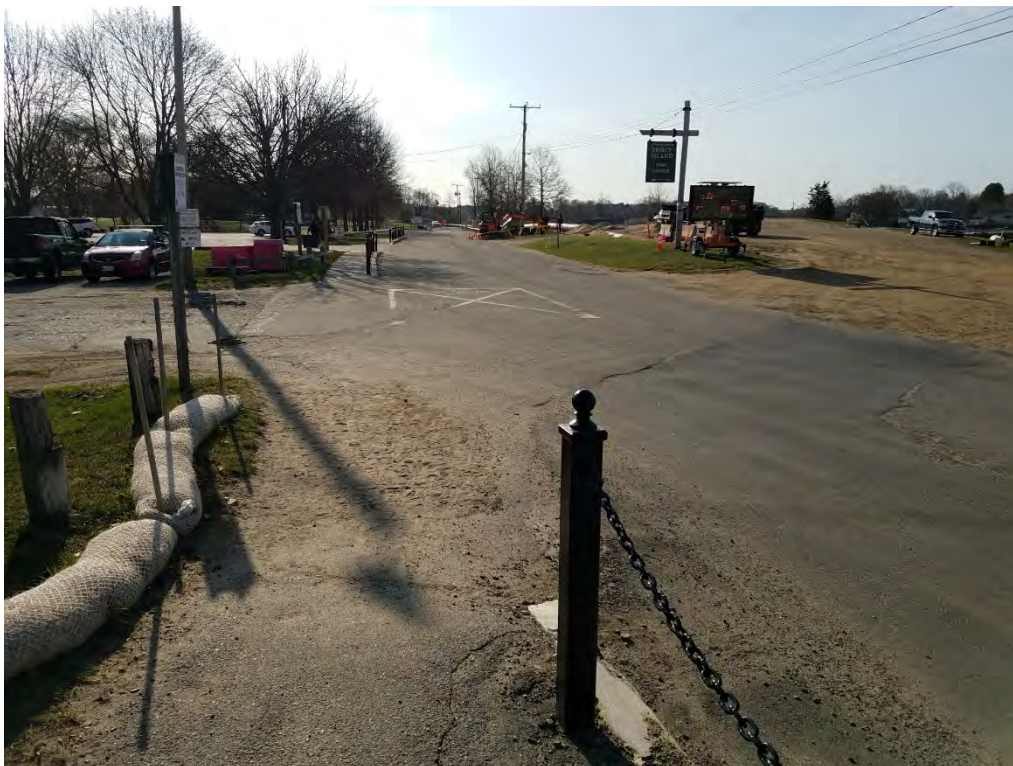
Photo 26. From the north side of the Peirce Island Bridge Rd. Bridge facing east. (04-15-21)
