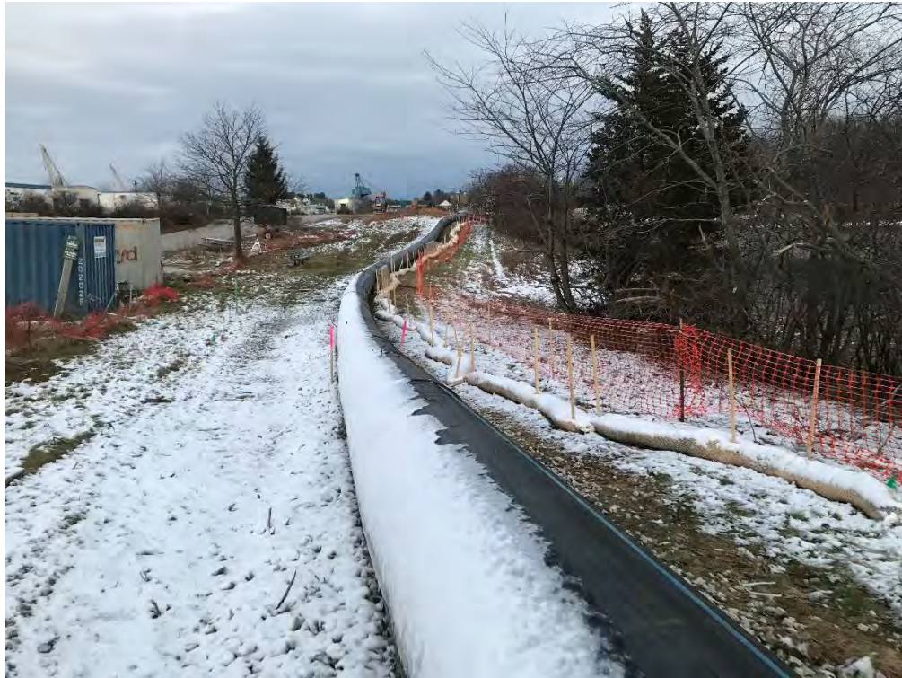
Photo 1: Construction Fencing Area A
