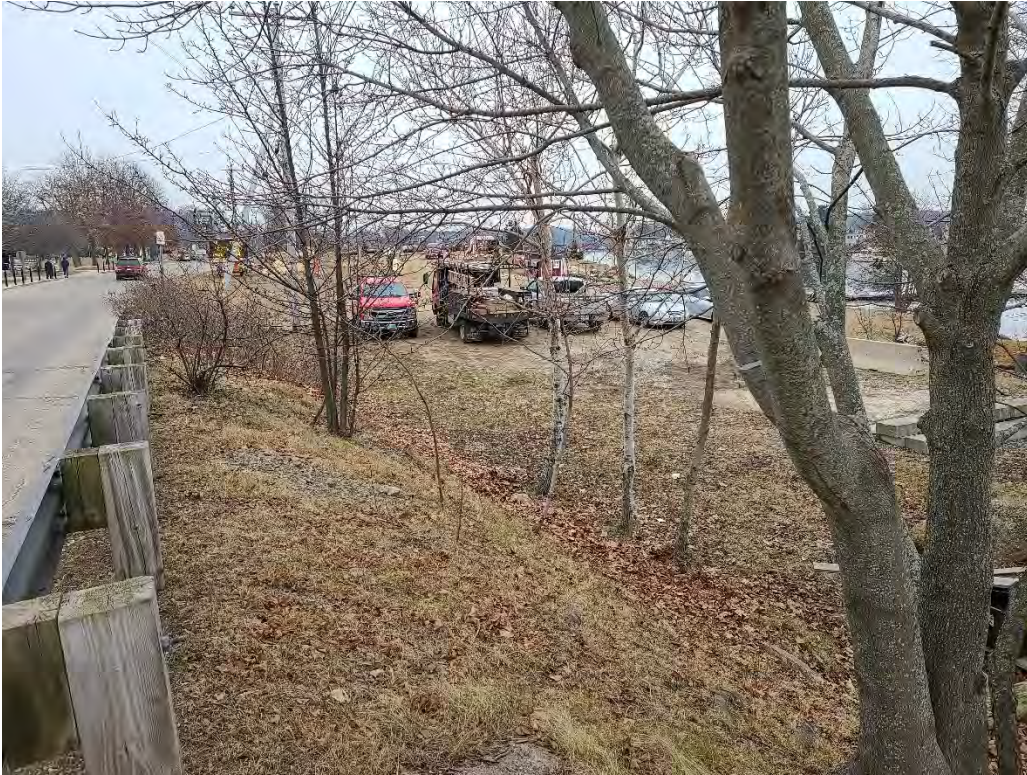
Photo 13. From bridge at western end of the pipeline replacement, looking east. (01-14-21)
