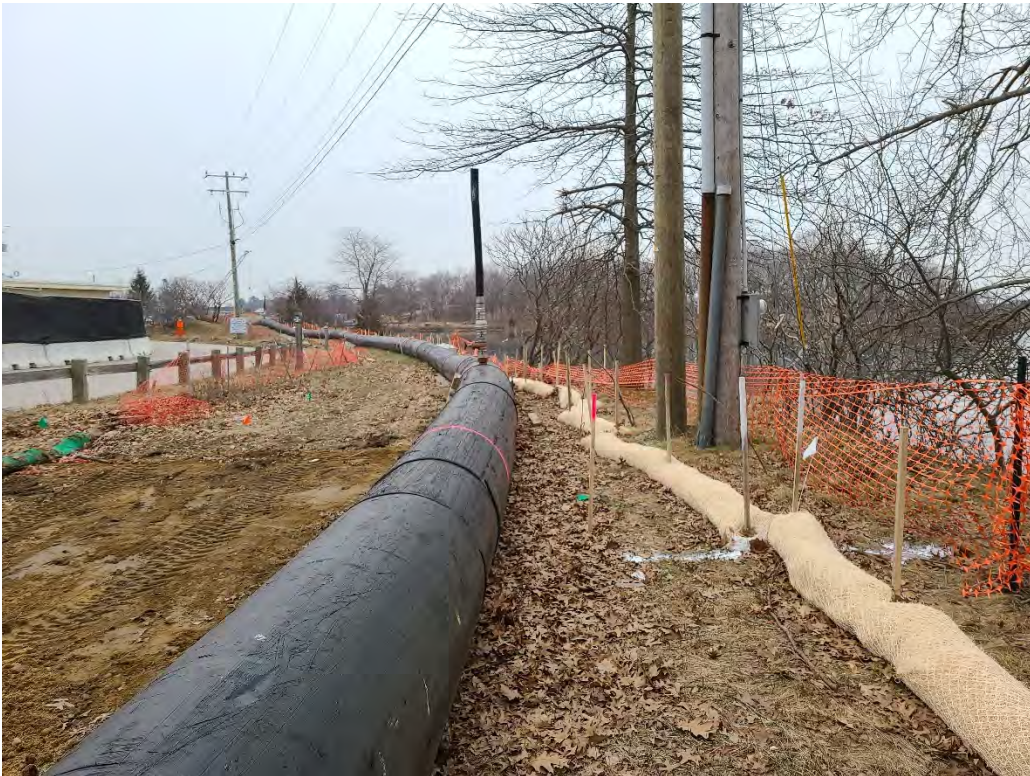
Photo 18. Along the pipeline replacement near Grid 46 of the tree inventory for the Pipeline Survey, looking east. (01-14-21)
