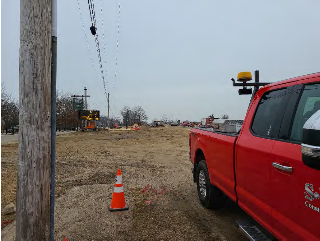
Photo 15. From the western end of the boat launch parking area along the pipeline replacement, looking east. (01-14-21)
