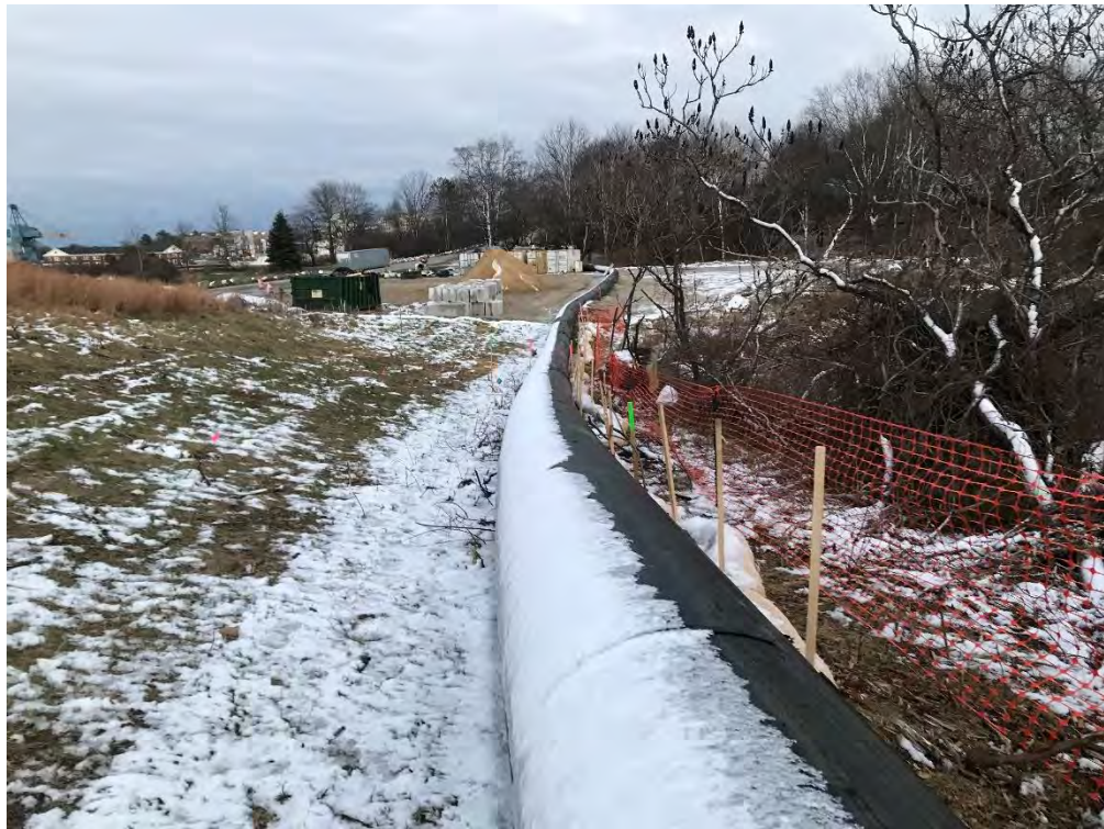
Photo 2: Construction Fencing Area B
