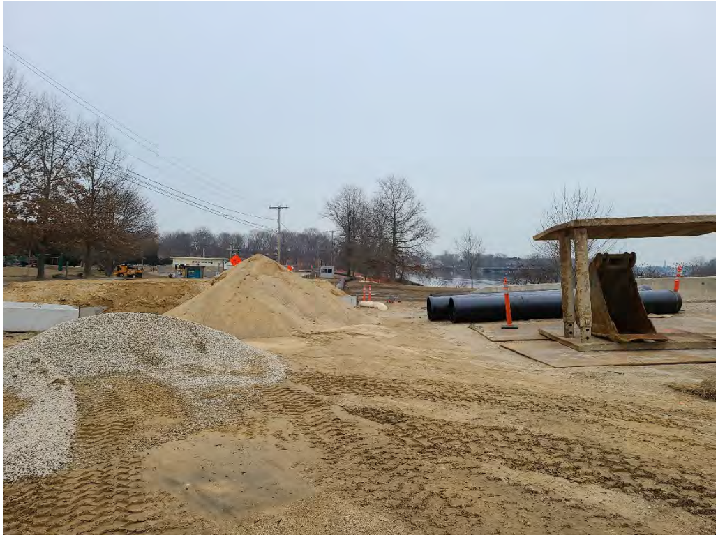
Photo 16. From laydown area at eastern end of the boat launch parking area, looking east. (01-14-21)
