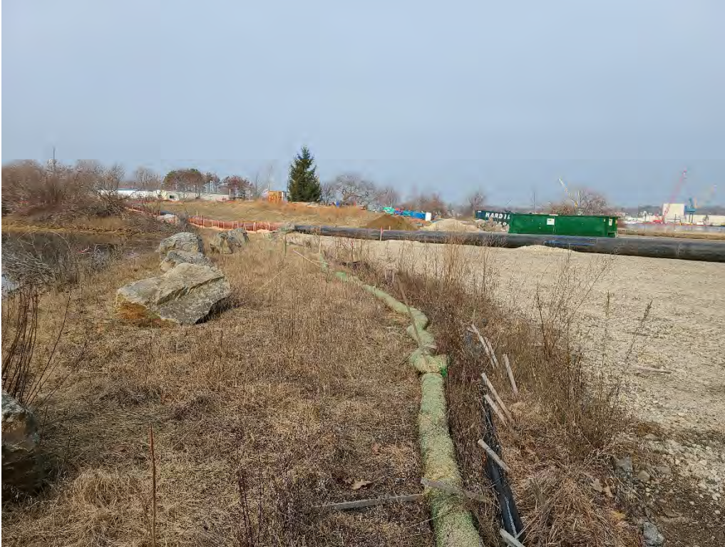
Photo 21. From eastern end of the pipeline replacement near the planned parking area, looking west. (01-14-21)
