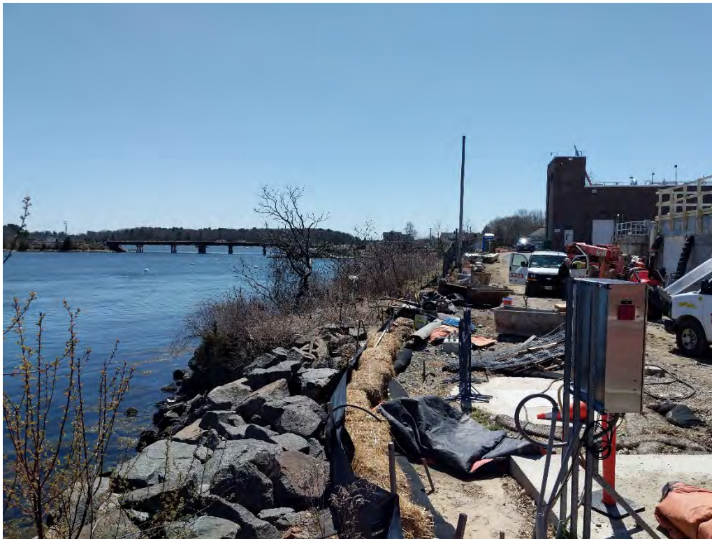
Photo 10. Rip-rap along the edge of the proposed path east of wastewater treatment facility, looking south. (04-23-20)
